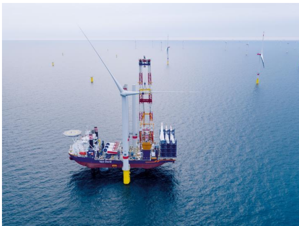
Figure 2.11: The AEOLUS jack-up vessel (JUV) from Van Oord installing a wind turbine (source Van Oord).
