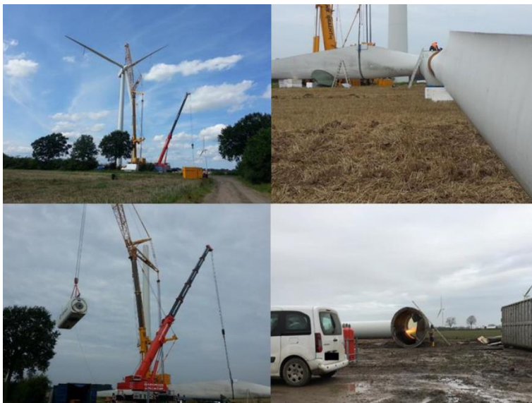
Figure 2.14: Decommissioning of an onshore wind turbine (source Ramboll [10]).
